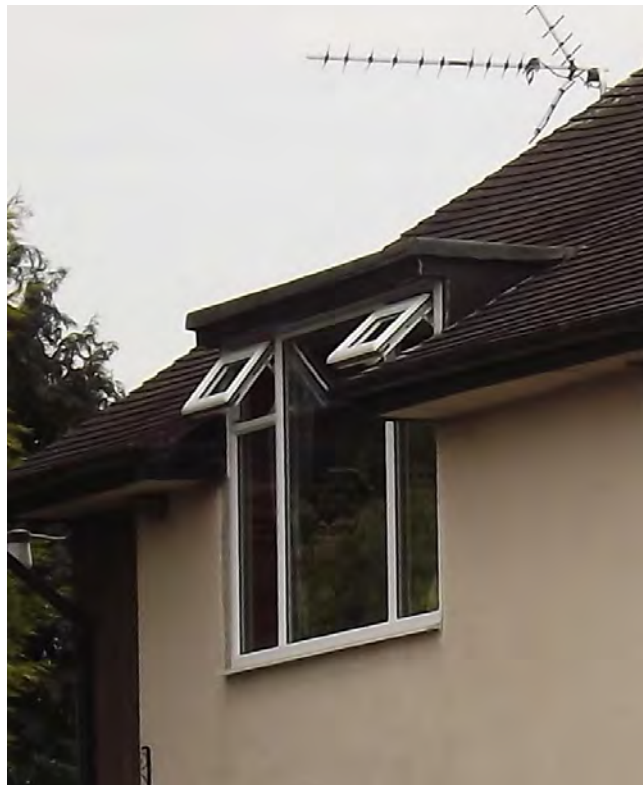
Figure 84 uPVC windows with horizontal openings are out of character with the conservation area
