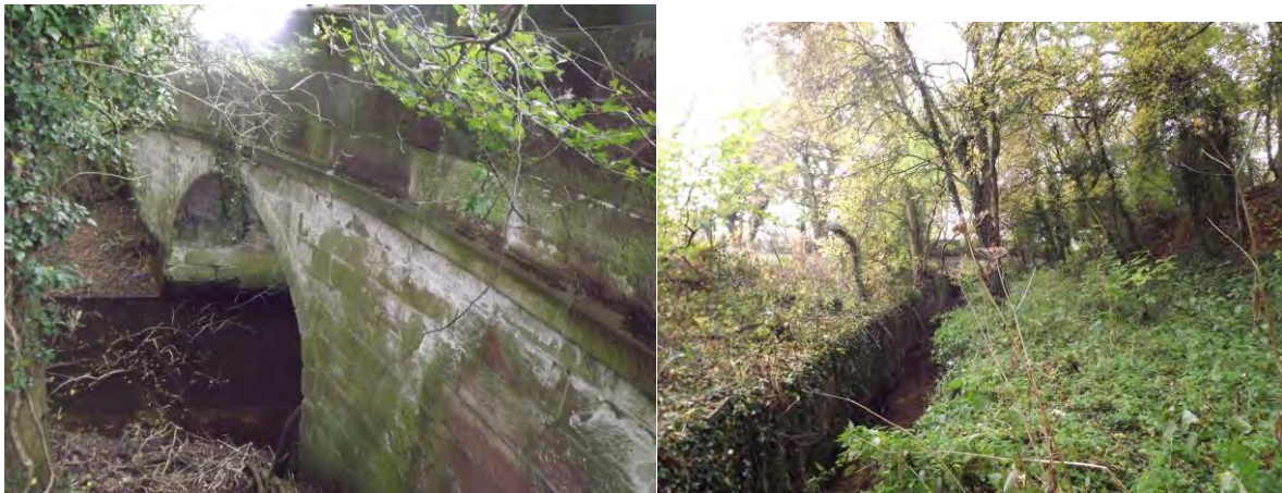
Figure 51 Oulton Bridge and lock chamber to lock no.7
