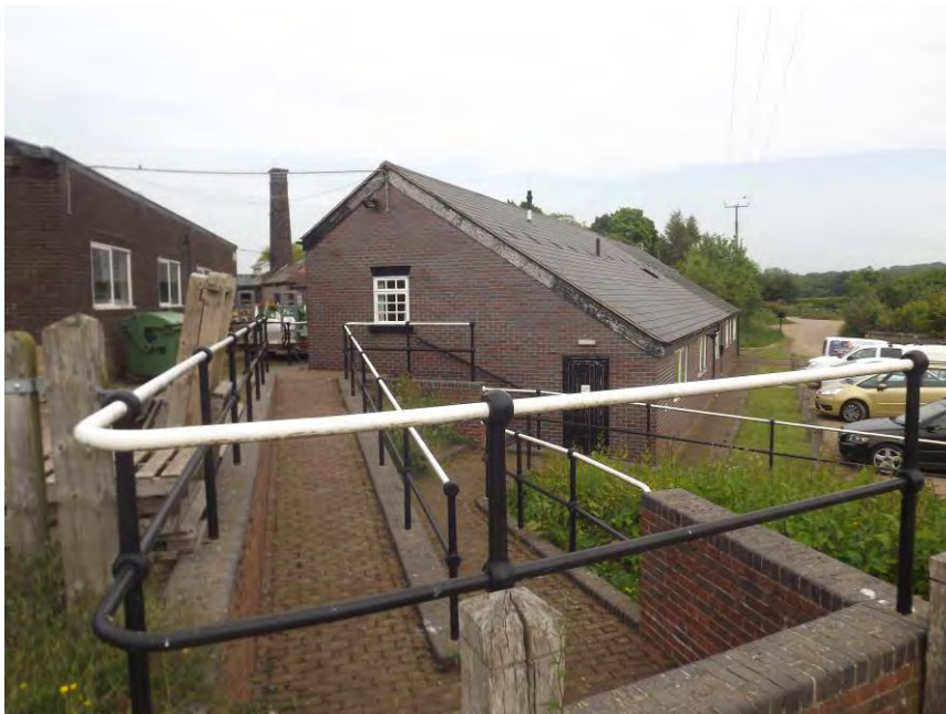
Figure 82 An extension to a maintenance yard building and modern railings is out of character with the conservation area
