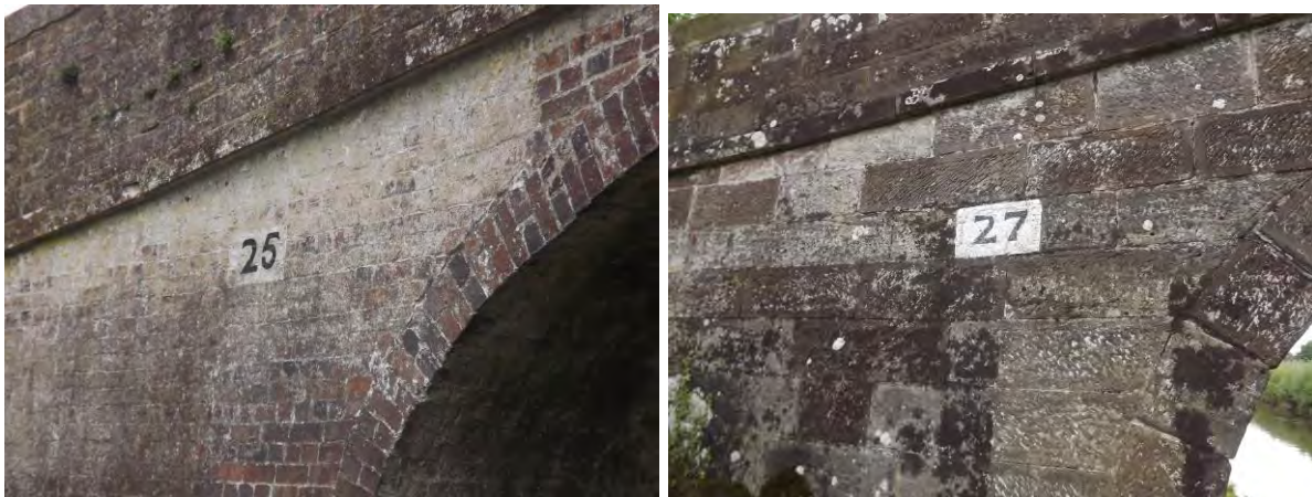
Figure 76 Painted bridge numbers are uncharacteristic
