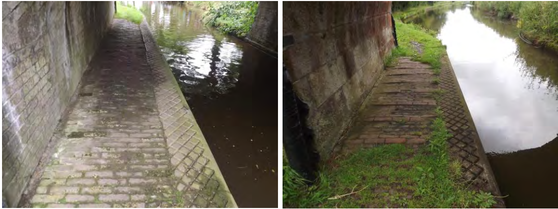
Figure 17 Examples of brick paving surfaces at bridges 26 and 27
