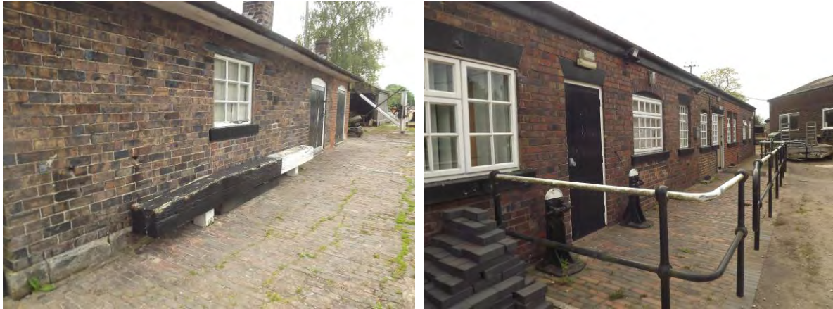
Figure 54 The former smithy and depot at the maintenance yard
