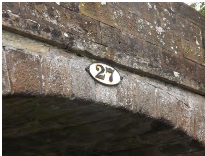
Figure 13 Cast iron bridge plates
