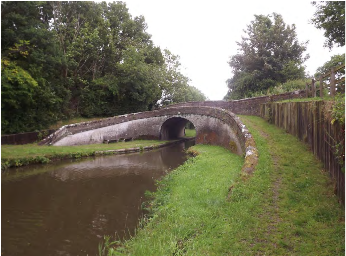
Figure 11 Roving Bridge no.26 north of High Onn Wharf
