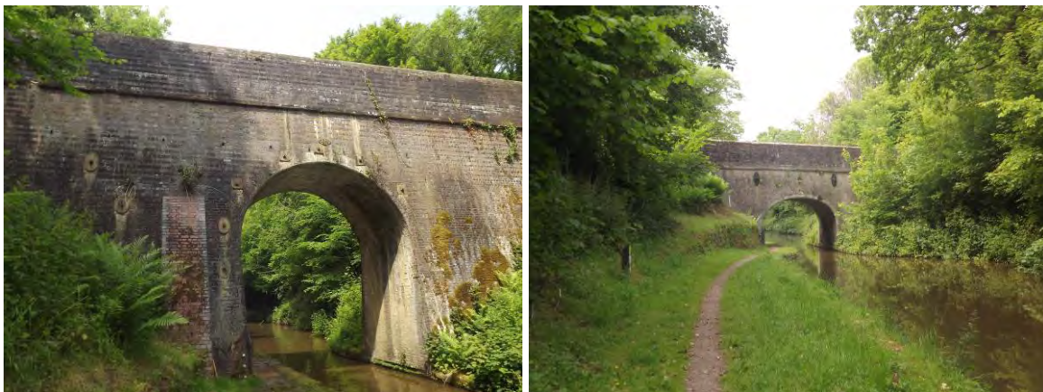
Figure 63 Double Culvert Bridge (No. 40) and Grub Street Bridge (No. 41)
