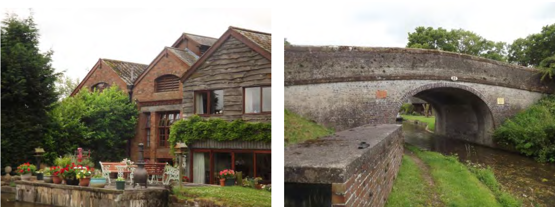
Figure 29 The former Cadburys milk processing building and High Onn Bridge
