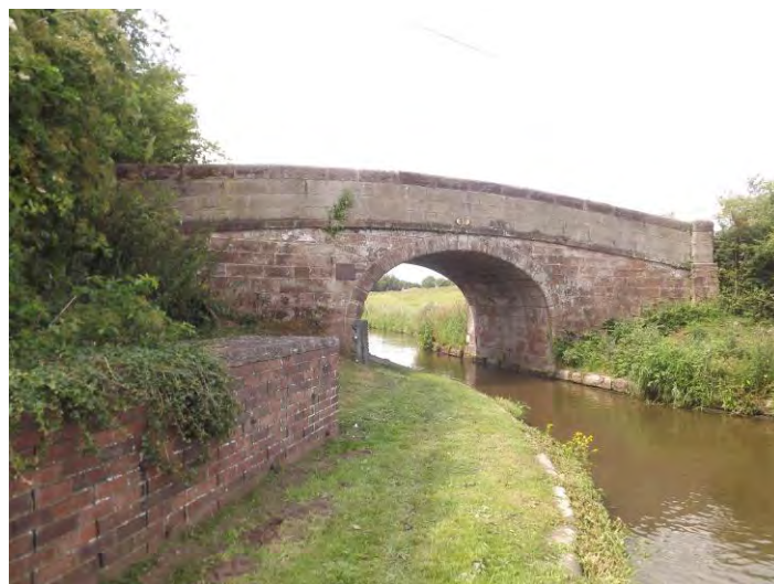
Figure 42 Machins Barn Bridge
