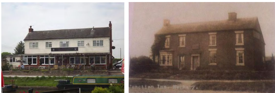
Figure 80 The Junction Inn today and prior to alteration in the early 1900s
