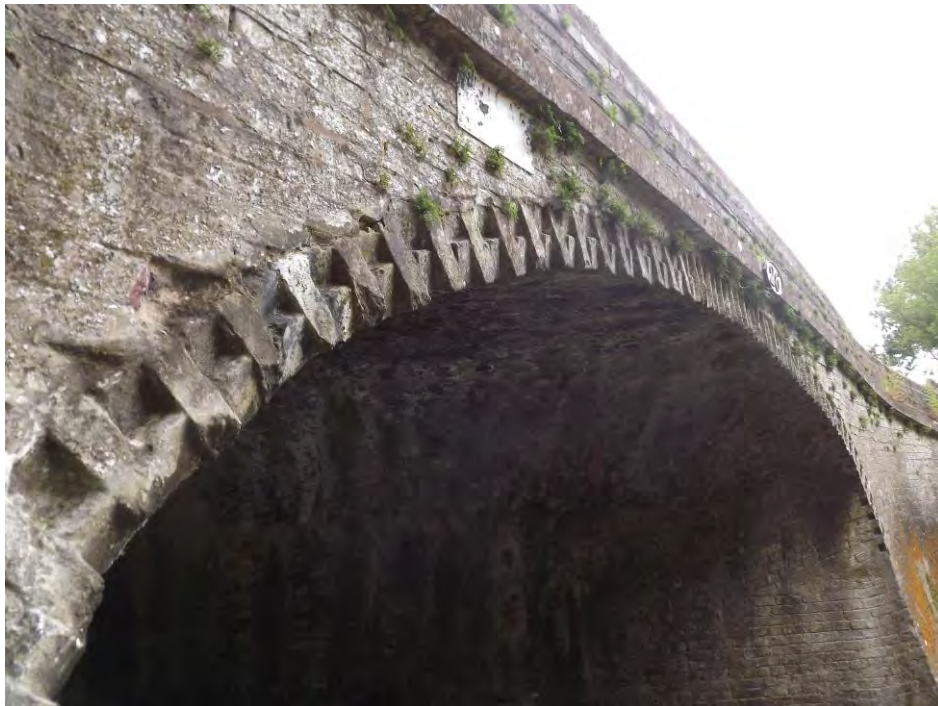
Figure 30 Brick detailing to Roving Bridge No.26
