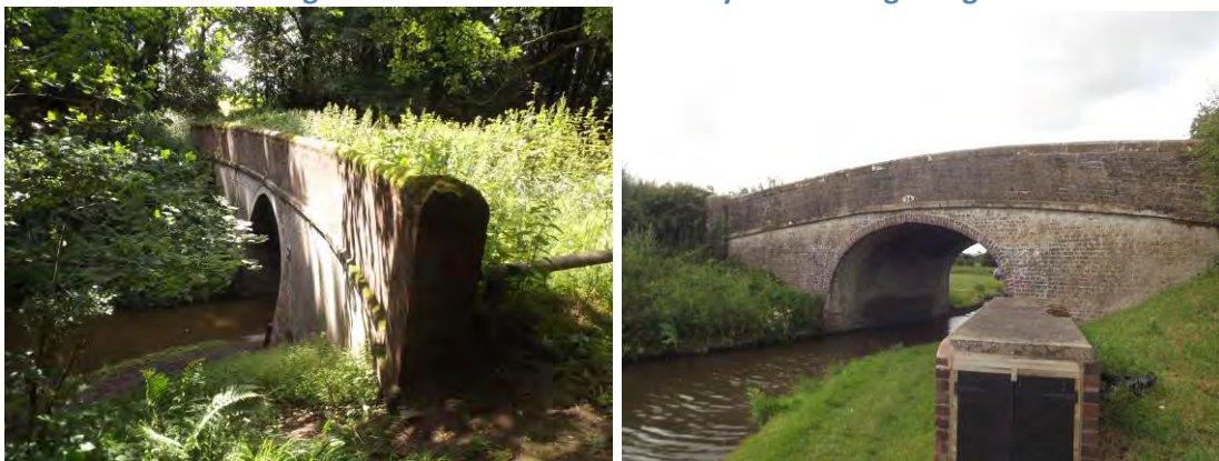
Figure 27 Ryehill Cutting Bridge and Little Onn Bridge
