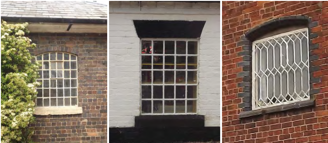
Figure 18 Multi-light, iron framed windows
