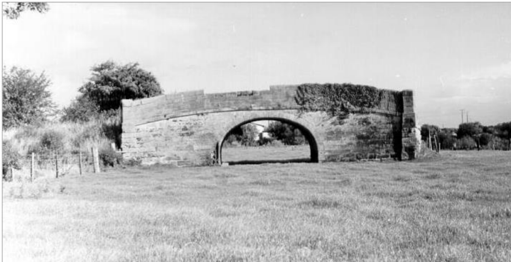
Figure 4 Blakemere Bridge (No.2) c.1980s a former accommodation Bridge on the Newport Branch
