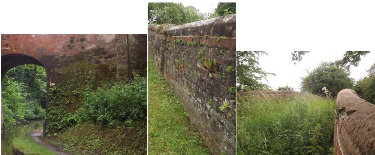
Figure 78 Vegetation growth to bridges can damage historic fabric and lead to structural problems
