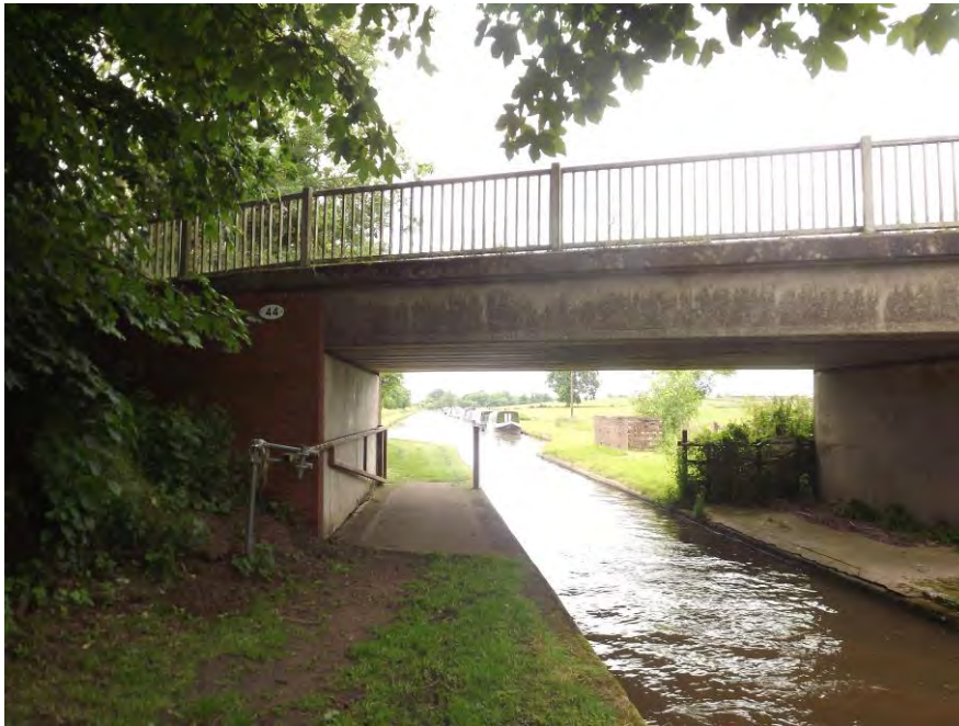
Figure 75 Shebdon Bridge no.44
