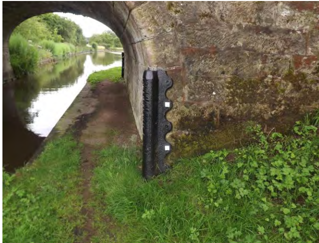
Figure 12 Iron strapping posts show evidence of tow rope wear
