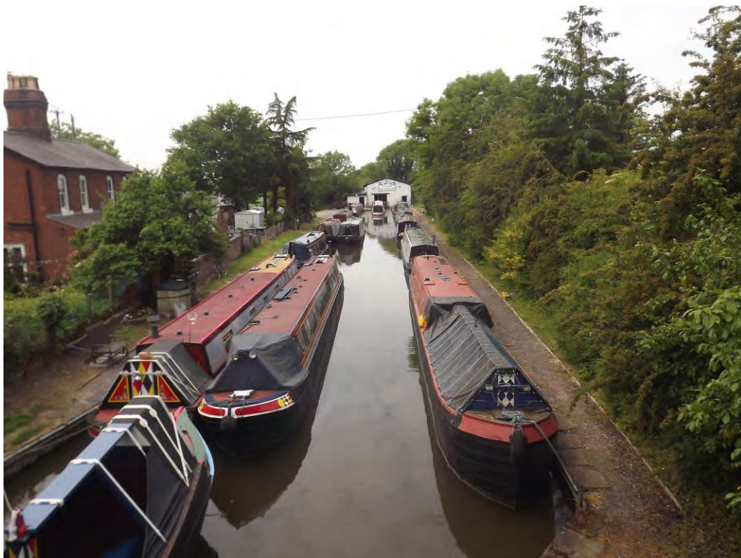
Figure 48 The junction of the Newport Branch with the Main Line of the Shropshire Union
