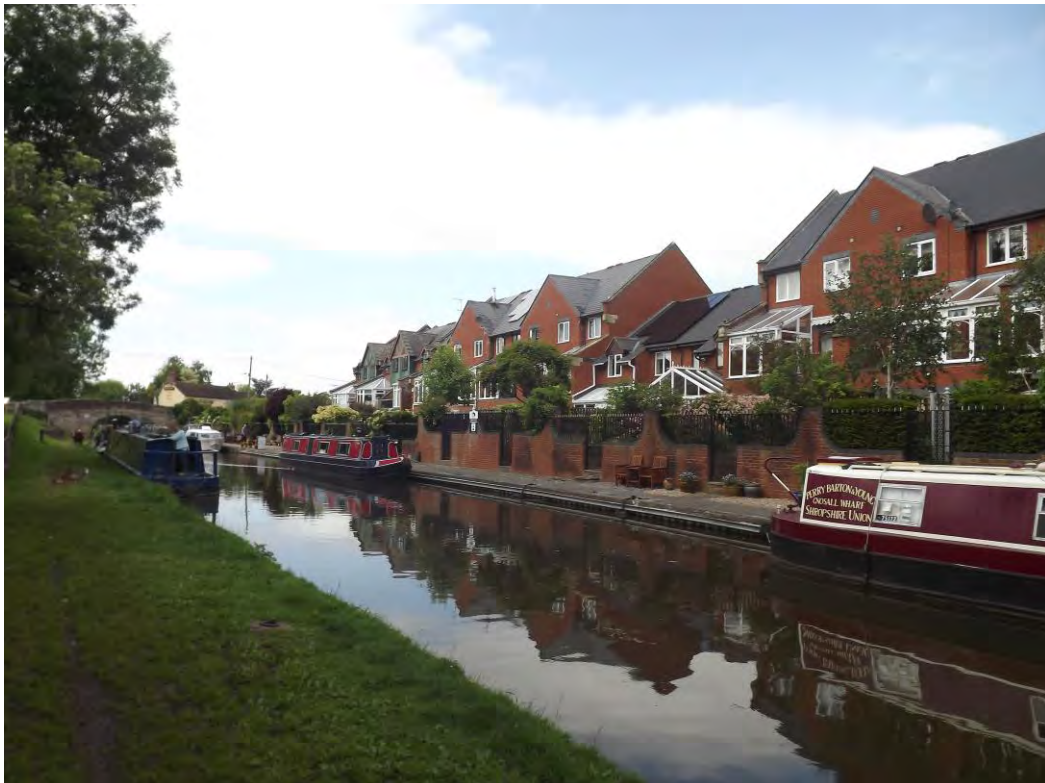
Figure 83 Modern canal side development can often dwarf smaller historic buildings and structures
