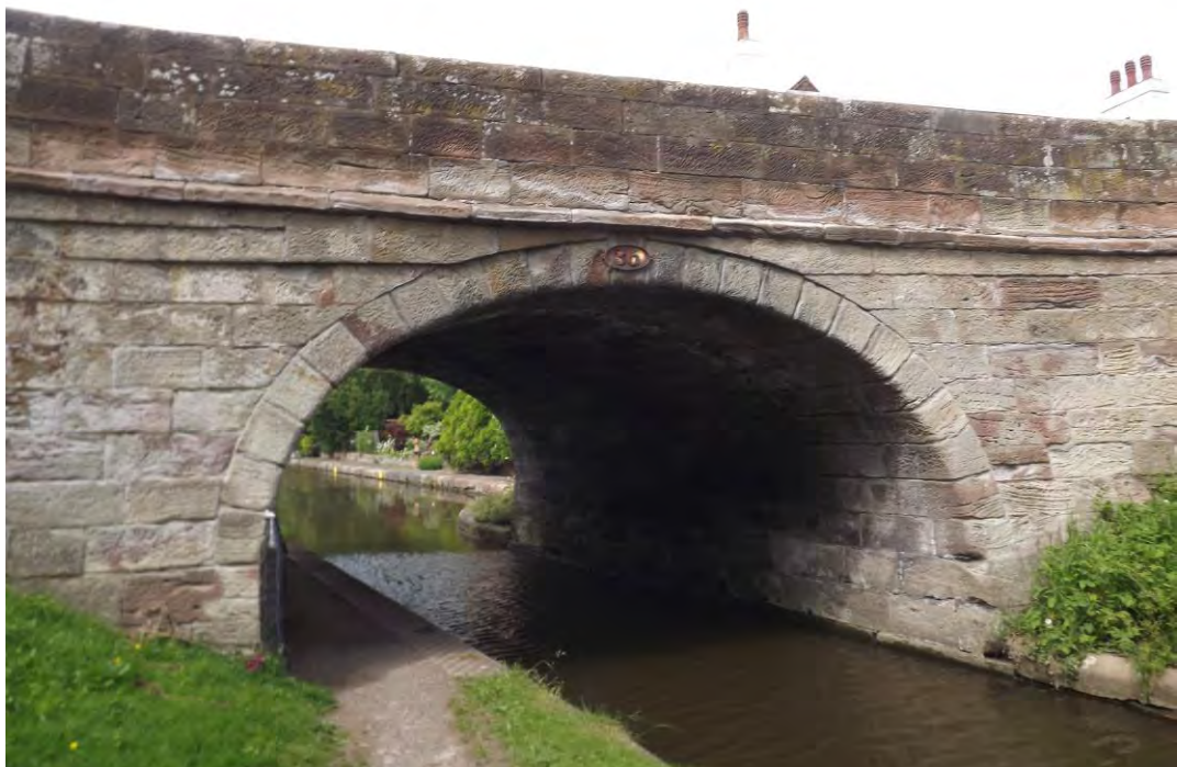
Figure 38 Newport Road Bridge
