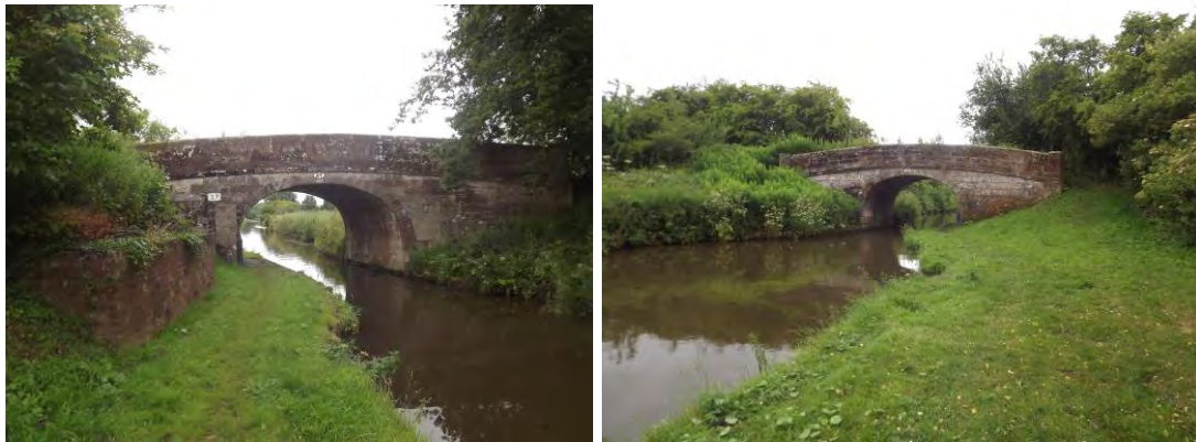
Figure 32 Parks Bridge No. 27 and Parks Barn Bridge No. 28
