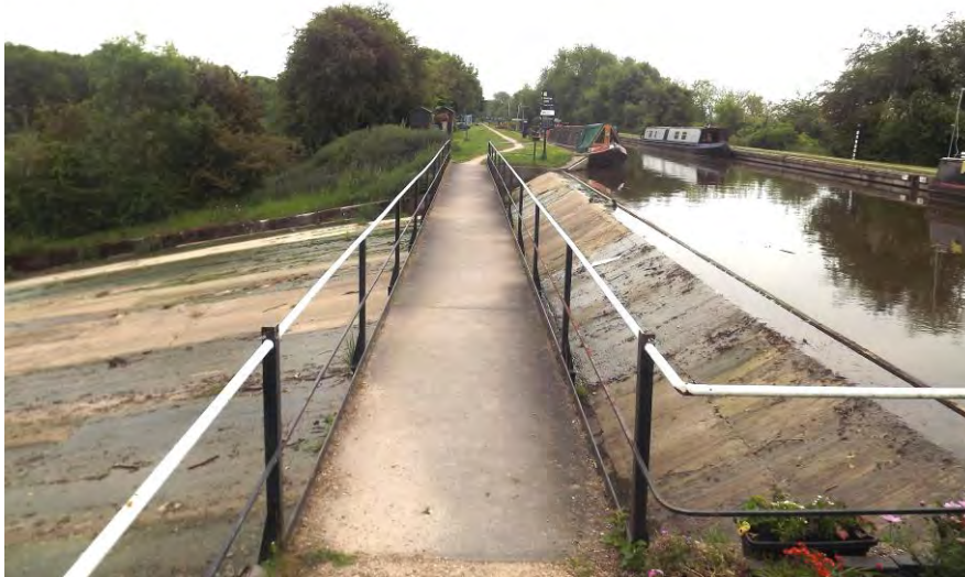
Figure 9 Sluice at Norbury Junction Wharf
