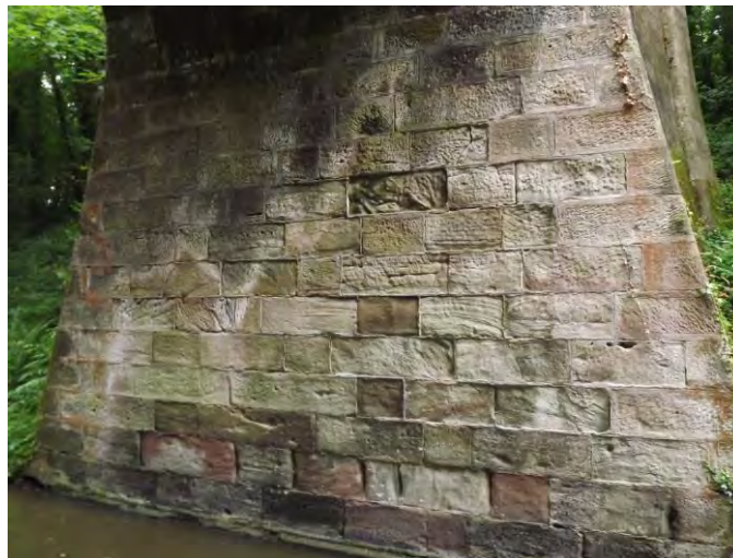
Figure 77 The use of cementitious materials can cause stone or brick to sacrificially decay
