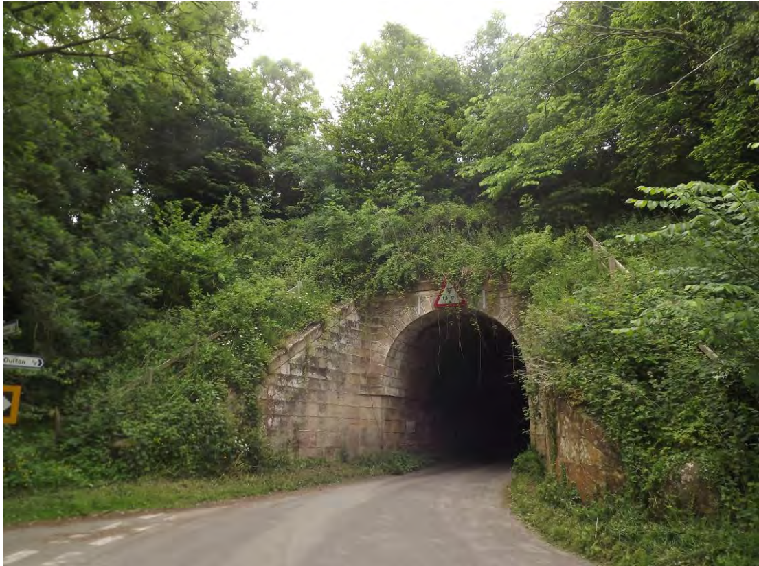
Figure 14 The grade II listed Shelmore aqueduct at the NW corner of Shelmore Wood
