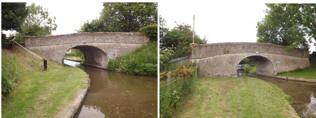
Figure 65 Old Lea Bridge No. 42 and Bullocks Bridge No.43
