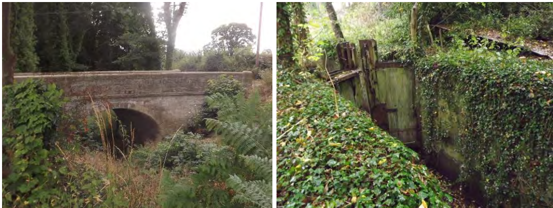
Figure 49 Parton's Bridge and lock chamber to former lock no.5
