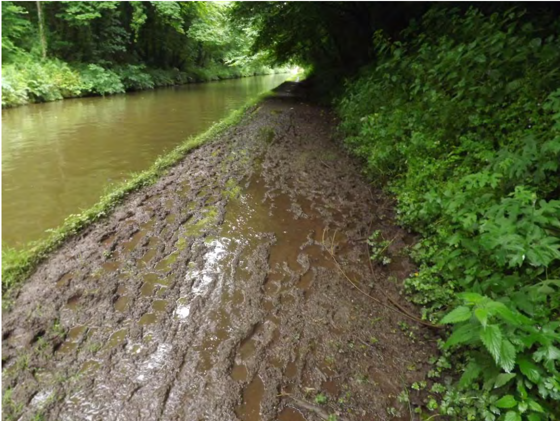
Figure 81 Some sections of tow path are excessively muddy making access difficult.
