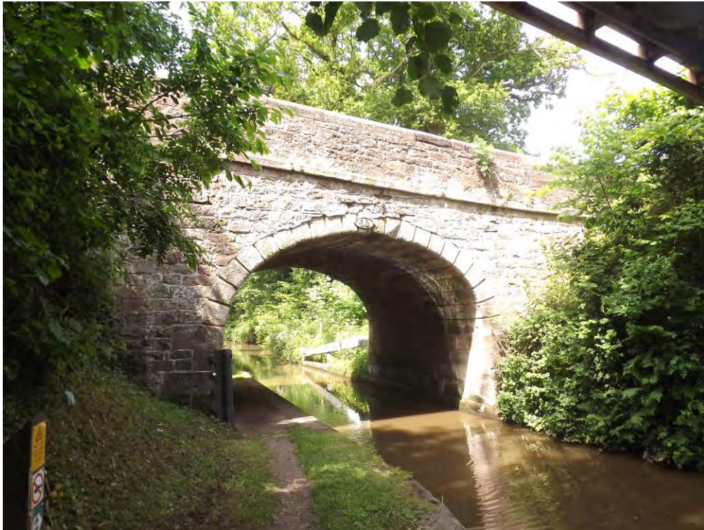
Figure 72 Newport Road Bridge
