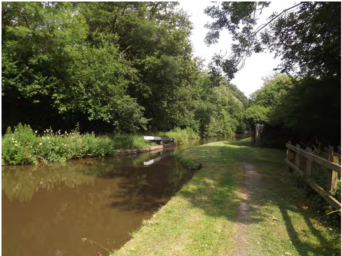
Figure 8 Stop gate at Shelmore Embankment
