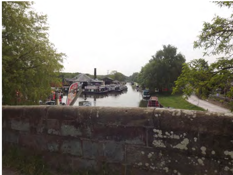
Figure 46 The wharf at Norbury Junction
