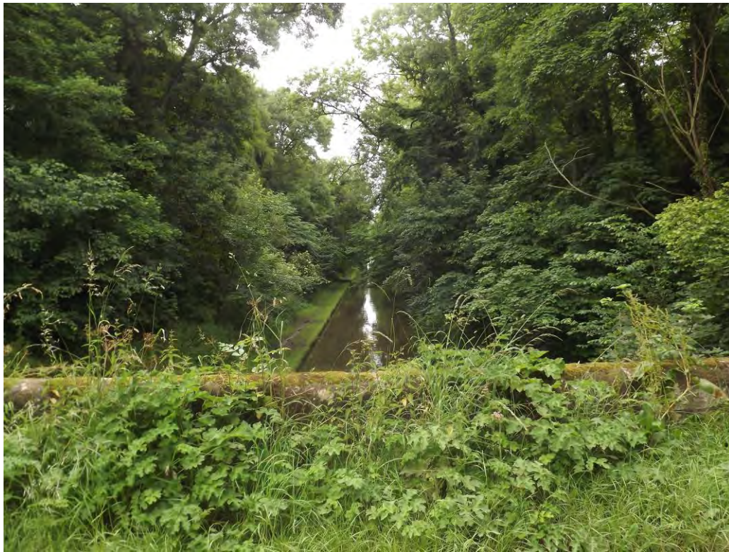
Figure 7 Heavily wooded cuttings are a feature of the Shropshire Union Canal- looking south from Wood Eaton Bridge
