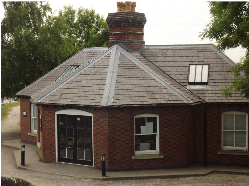
Figure 86 The Canal and River Trust headquarters at Norbury Junction reflects the hipped and octagonal roof styles of the lock keepers cottage
