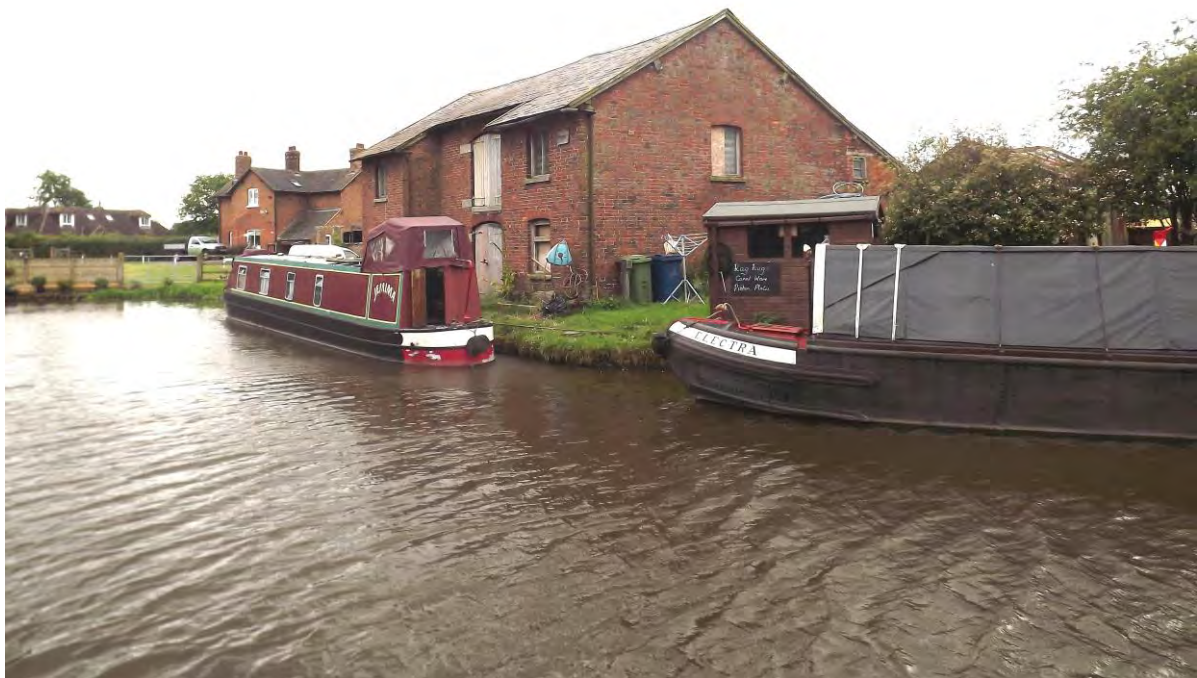
Figure 22 Warehouse at High Onn Wharf
