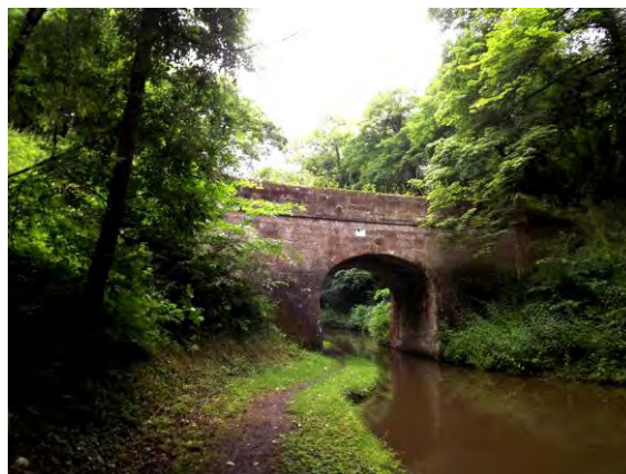
Figure 33 Wood Eaton Bridge marks the entrance to Castle Cutting
