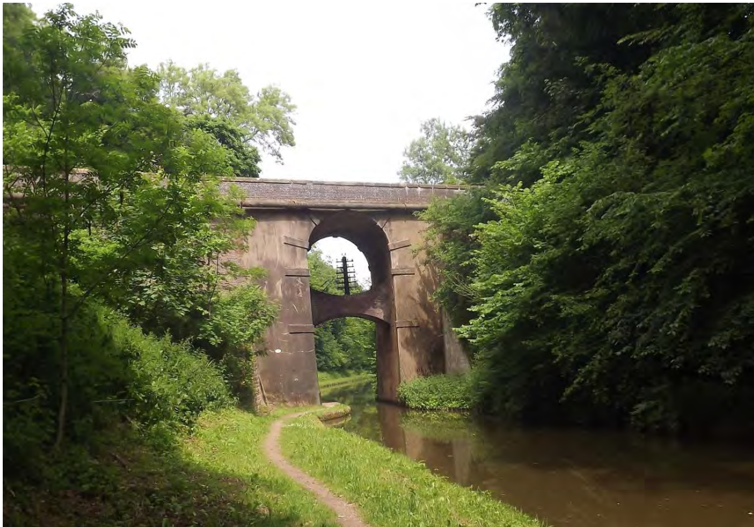
Figure 10 High Bridge (39) displays an unusual double arch
