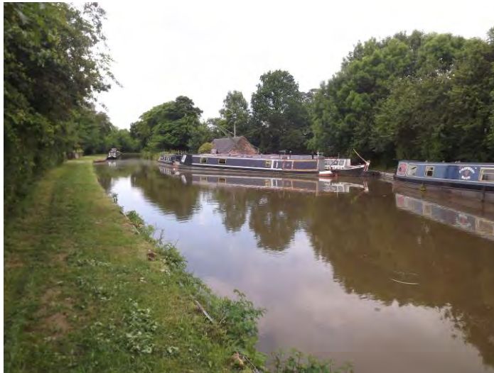
Figure 68 Shebdon Wharf and winding hole
