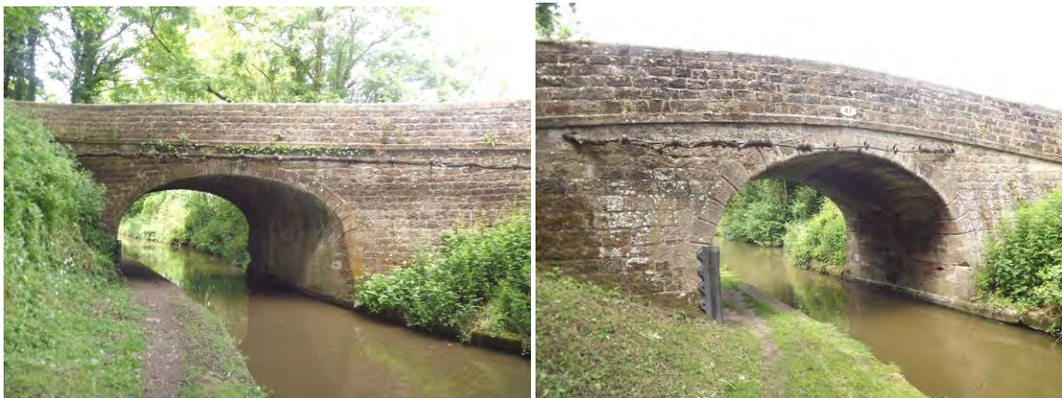
Figure 73 Knighton Bridge and Black Flats Bridge
